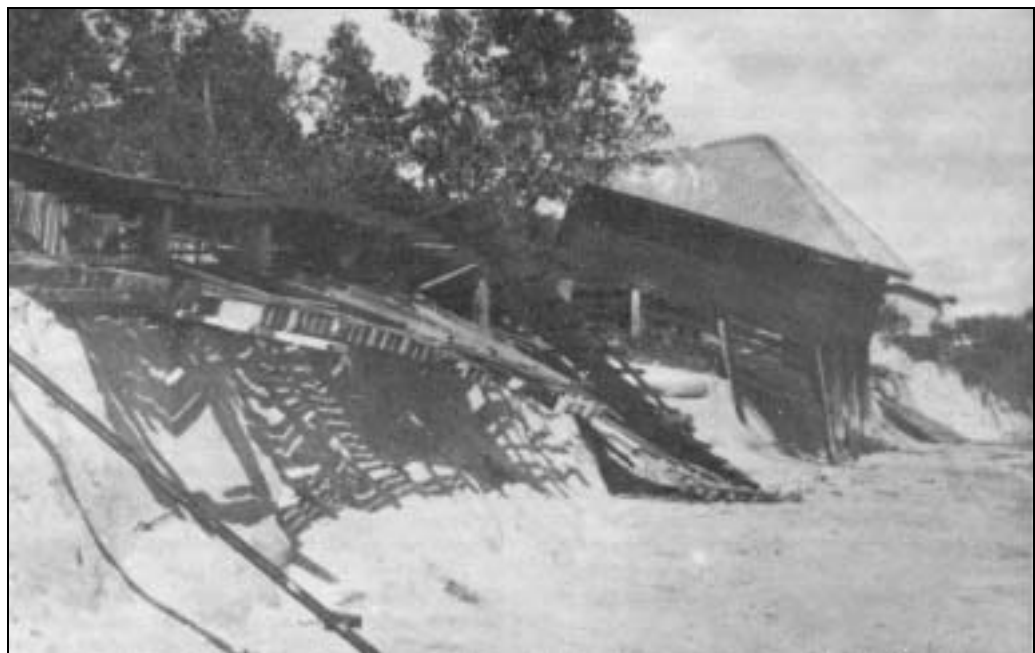
Figure 5. Dressing sheds on Main Beach falling into the sea as a result of the 1947–48 cyclones (Source unknown)
